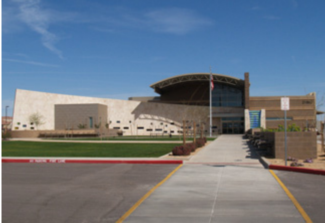
The Community Library and Recreation Center in Queen Creek, Arizona, has an energy efficient McQuay Modular Central Plant that contributed points toward LEED® Gold certification for the building.
