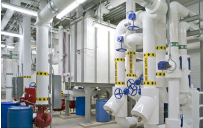
Applied Development Center—Interior, Plymouth, MN
